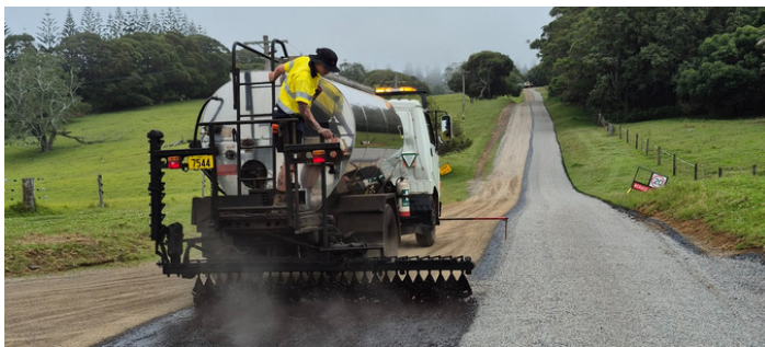
Calebs Lane during reconstruction works
