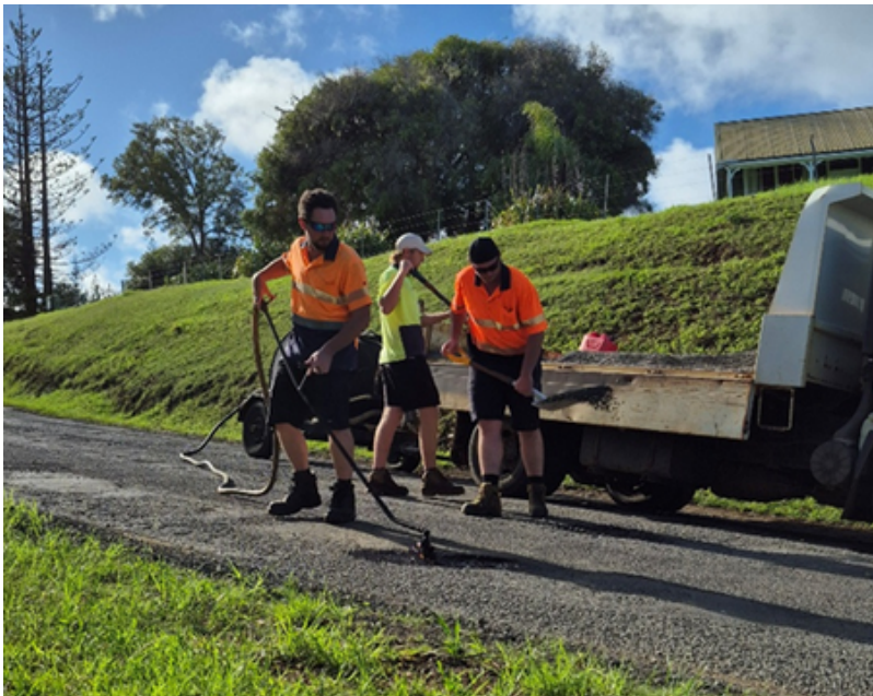
Image: Pothole patching
