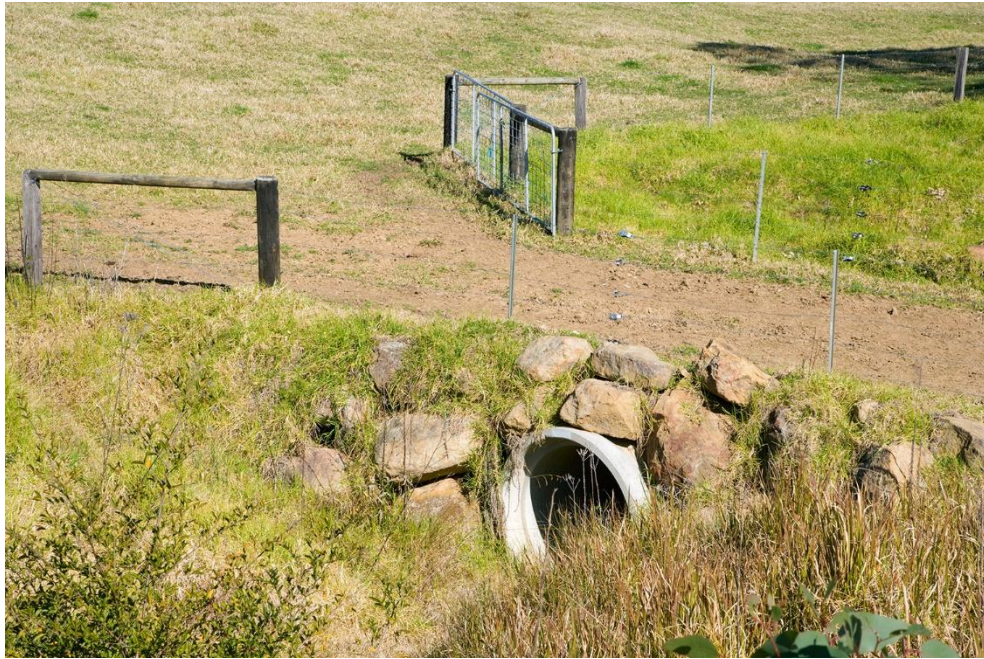
Image 4: Stabilised, fenced culvert crossing with hardened approaches and protected banks to concentrate stock access and minimise erosion and direct waterway disturbance. Source: Stock & Waterways (2019). Photo: Stuart Naylor.
