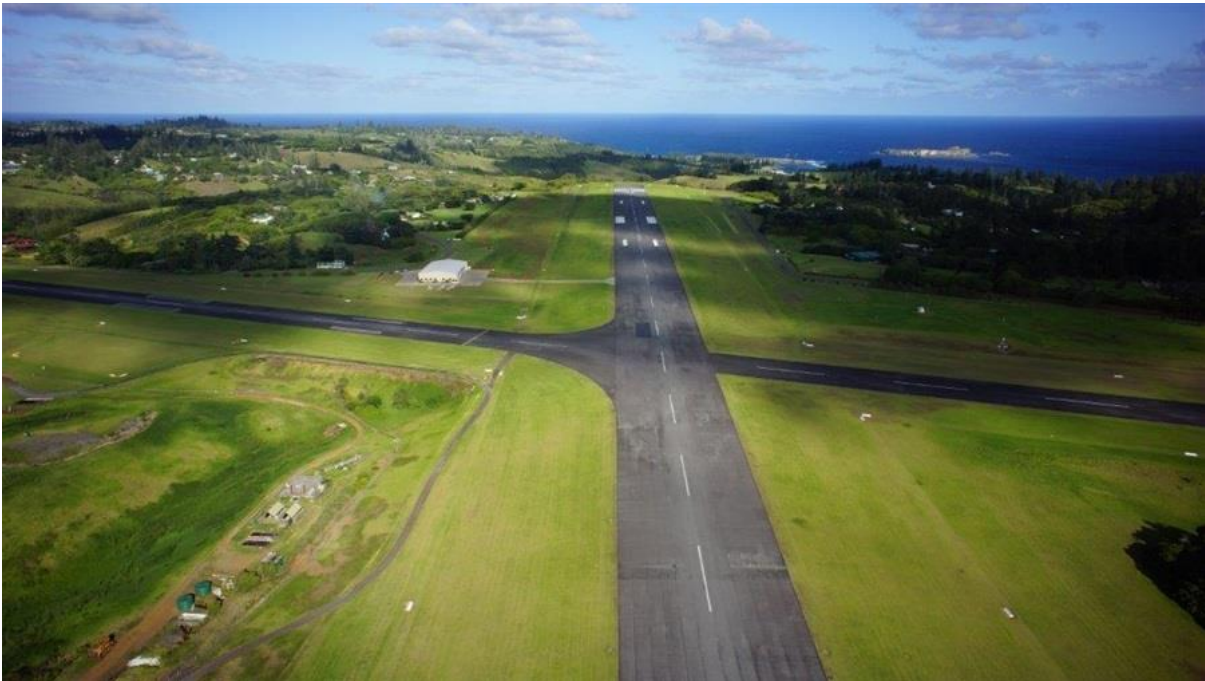
NORFOLK ISLAND AIRPORT RUNWAYS AND SURROUNDS
