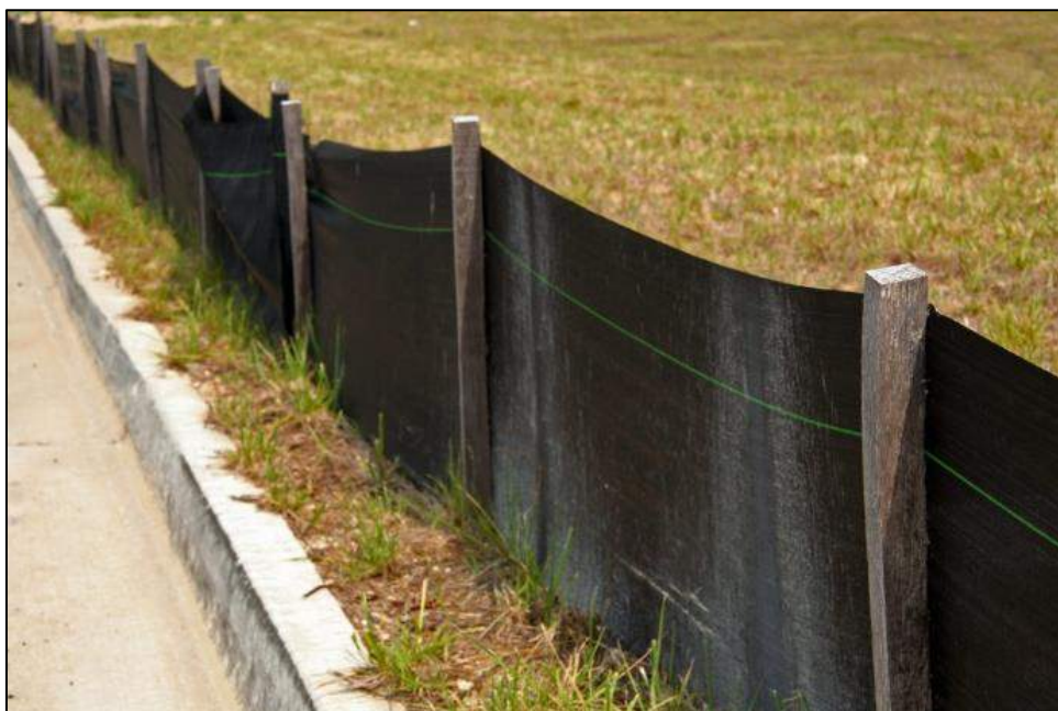
Figure 9.3: Example of Silt Fence in a Road Verge
