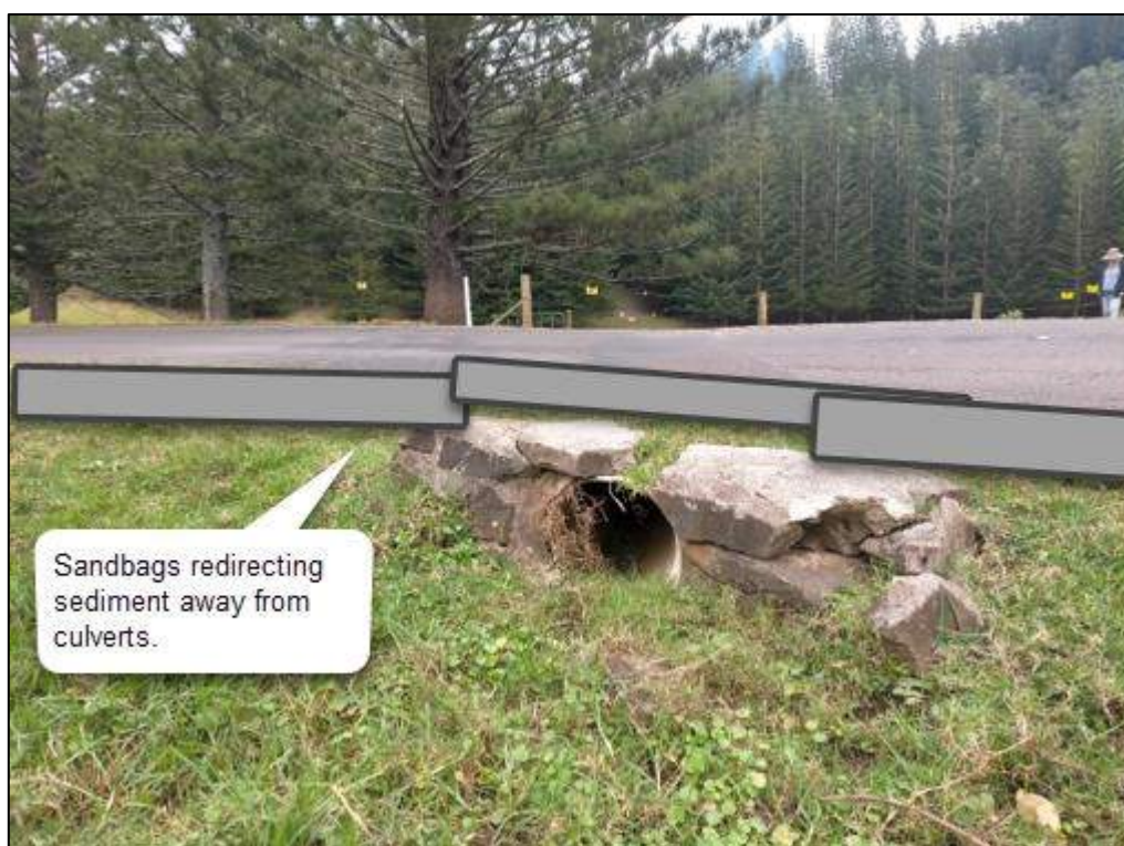
Figure 9.7: Example of Culvert and Sandbags
