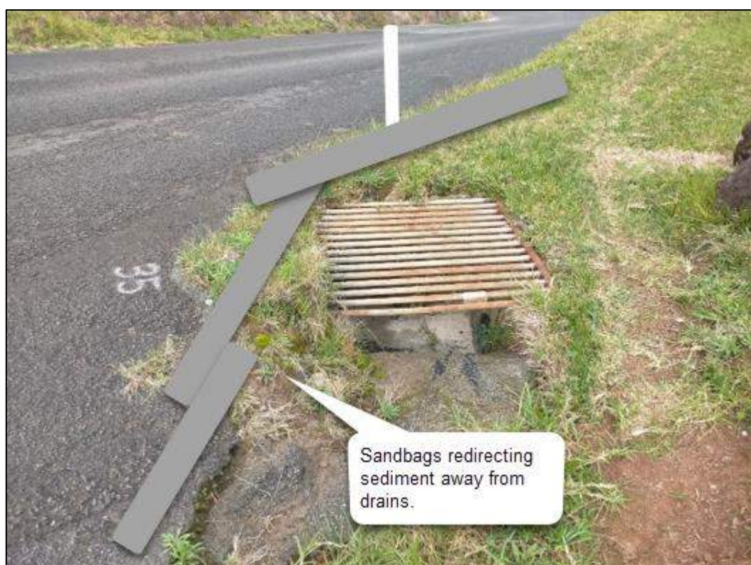
Figure 9.8: Grated Drain and Sandbags
