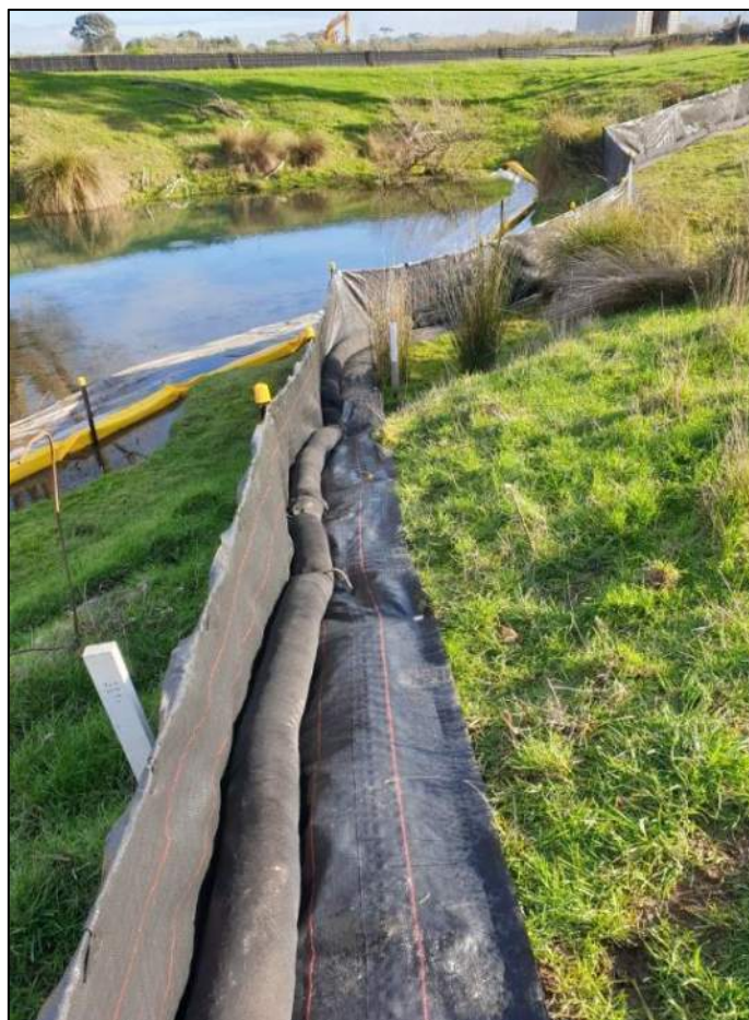
Figure 9.6: Example of Silt Fence combined Sandbag Erosion Protection Barrier
