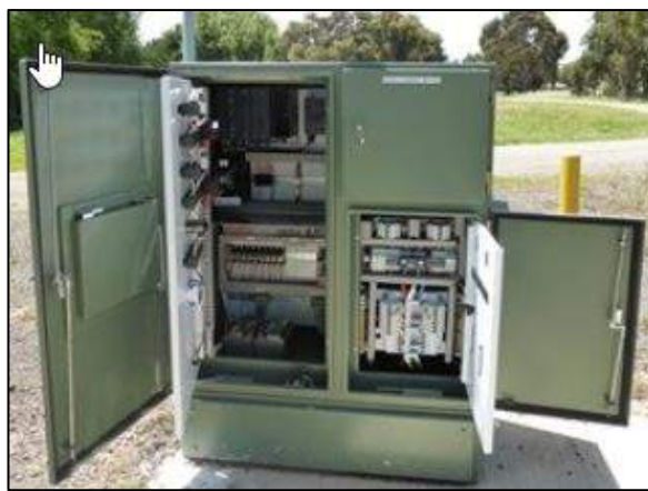
Figure 6.7: Typical Wastewater PS Control Cabinet
