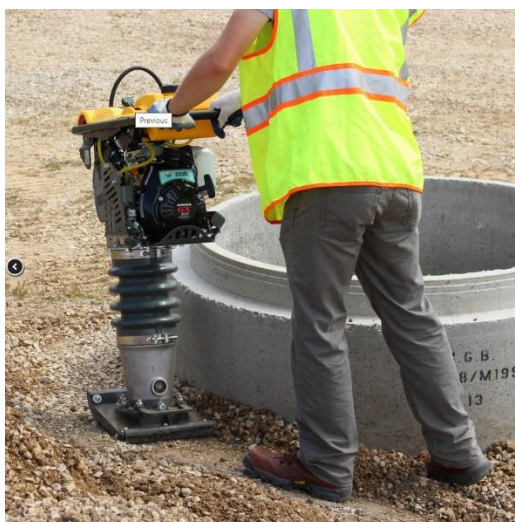
Figure 7.5-1: Wacker Neuson BS65-4As vibrator rammer
