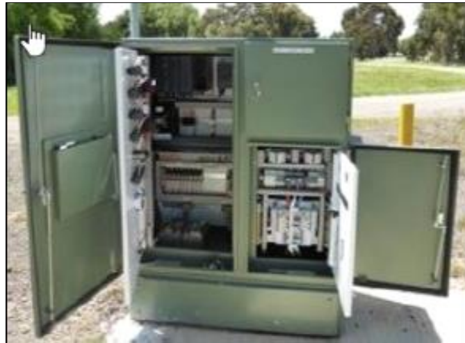
Figure 7.7-2: Typical sewage pumping station control cabinet (Source: Fluent Solutions, 2023 ( Appendix C ))
