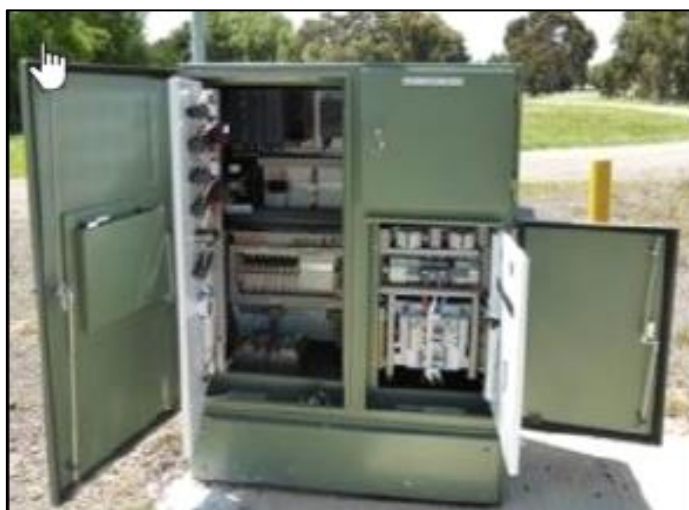
Figure 4-6: Typical sewage pumping station control cabinet
