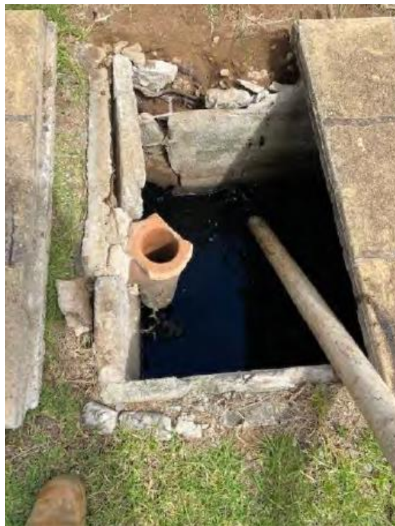
Figure 2-2: Example of a defective sewage holding tank in KAVHA prior to interim remediation work
