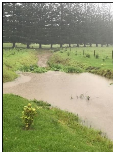
Figure 2-4: Leaky weir in operation
